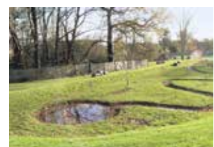
Attenuation ponds retain run-off and remove contaminants before draining into a water course.
